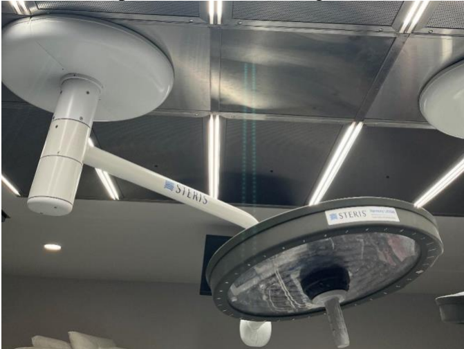
An overhead light in a resource-rich setting with multiple LED bulbs and a sterilizable handle that allows the surgeon to adjust and direct it.
