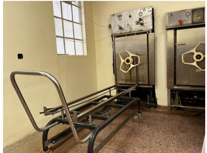
Wall-mounted autoclaves in the sterilization area, with a trolley to support the rack as it is being unloaded.
